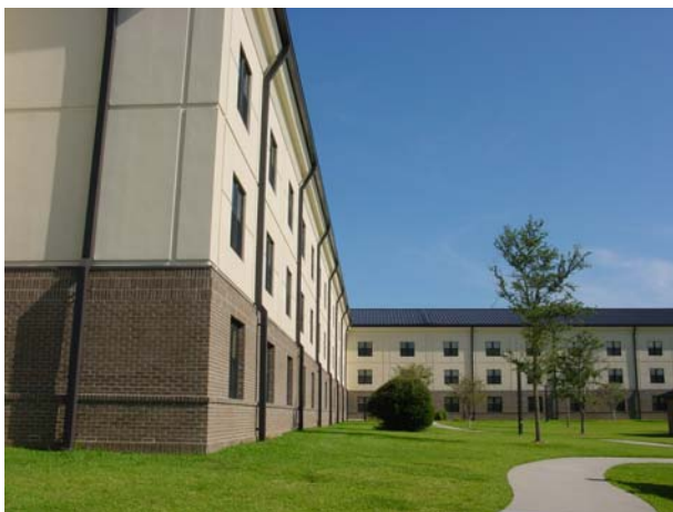
Kessler Air Force Base – Pipeline Dormitory
