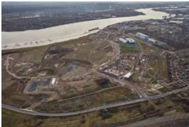
Barking Riverside before...
